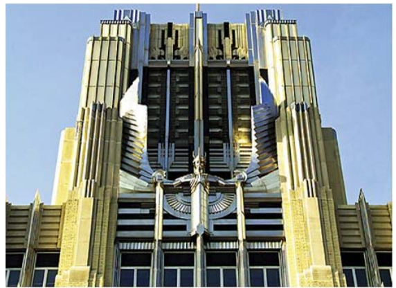
Architettura orwelliana. Niagara Mohawk Building. Syracuse, NY.
